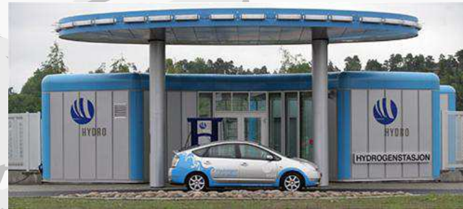
Hydrogen fueling stations
